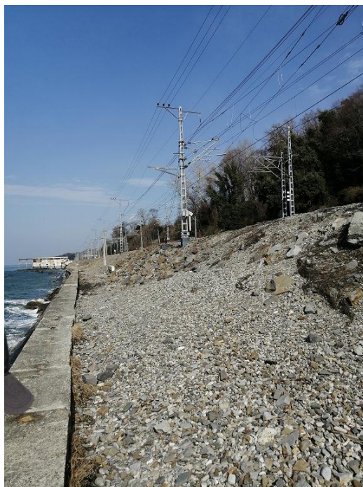
Figure 9. Railway line along the Black Sea coast between Tuapse and Adler (Photo by Mikhail A. Scheglov)
