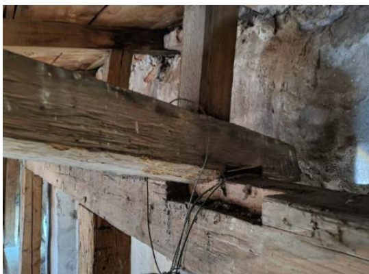
Fig. 4 Twisting of a Rafter's Cross-Section
