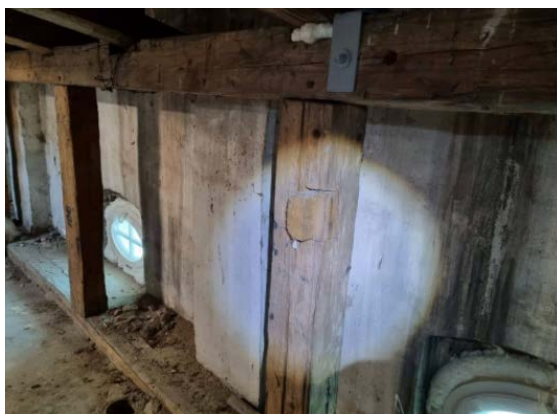
Fig. 5 Removal of an Original Structural Element
