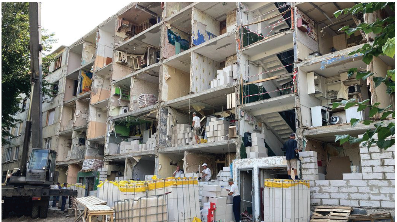
Fig. 5 The repair process of a large-panel building (sources: Information at https://cdn4.suspilne.media/images/resize/1040x1.78/680874f014cfdd08.jpg )
