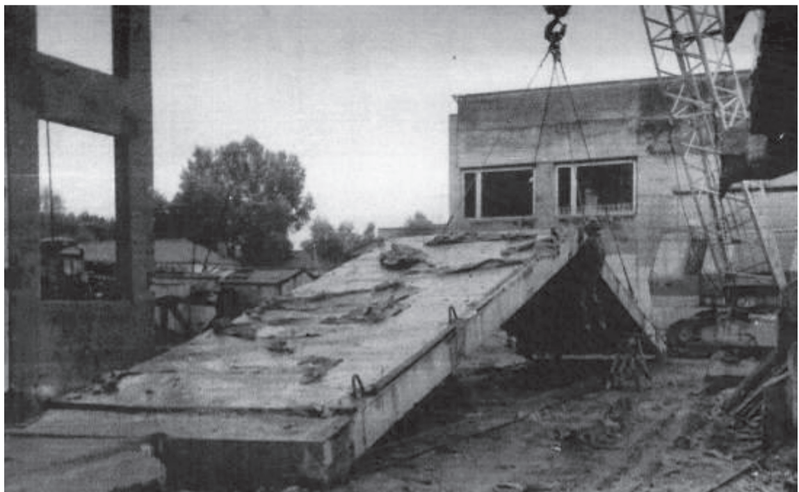
Fig. 5 Enlarging assembly of the covering panel and tensioning of the brace on the construction site
