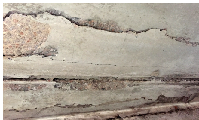
Fig. 3 An area showing the falling off of the surface layer of the concrete (part of the concrete layer is hanging down), S_{\text{area}} = 0.32 m 2 (pink color of concrete). The crack in the protective layer of the concrete has a length of l = 1440 mm and a width of a = 2.6 mm
