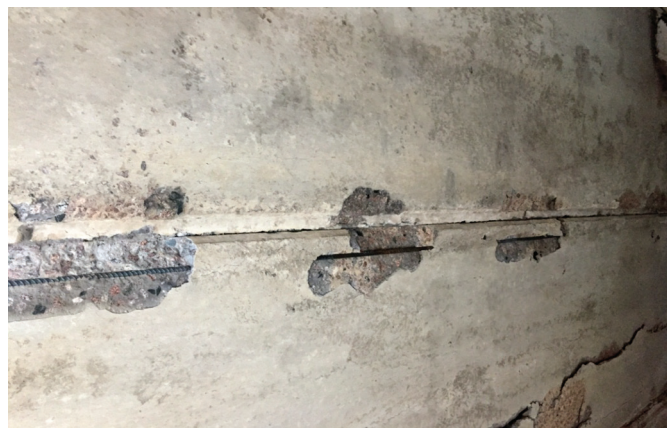
Fig. 4 Areas showing the destruction of the protective layer of the concrete, S_{area} = 0.04, 0.07 and 0.065 \text{ m}^2 , respectively, and the exposure of the working reinforcement (in the middle section, there are traces of soot on the reinforcement)
