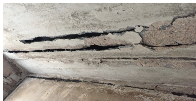
Fig. 1 Two sections showing the complete destruction of the protective layer of concrete with a length of l = 2400 \times 1360 mm and a width of a = 77 \times 72 mm, respectively
