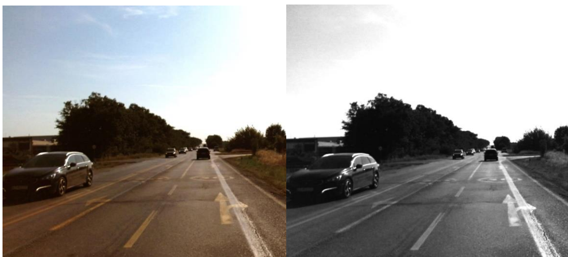
Figure 5: Outdated temporary lane markings on the road I/61 (color and grayscale).
