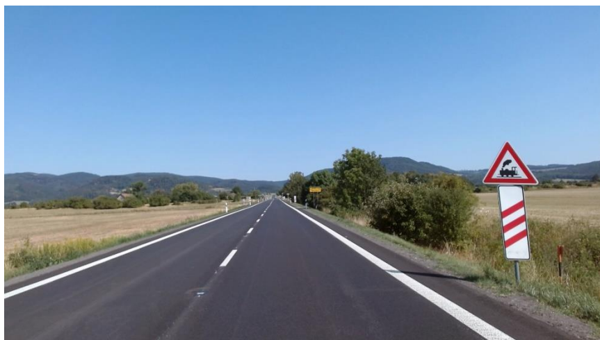
Figure 2: Ideal situation – newly reconstructed road II/503.
