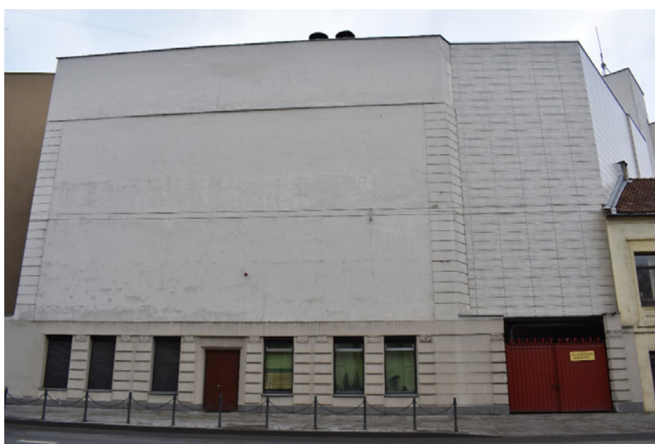
Fig. 5. The building at E. Ožėškienės Street, 13, which was demonstrated in the experiment
