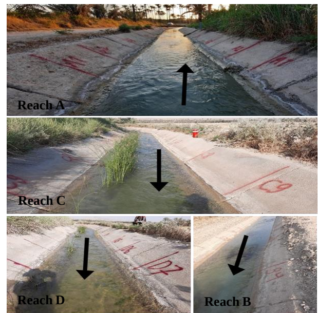
Fig. 2. Pictures of the selected reaches and measured sections
