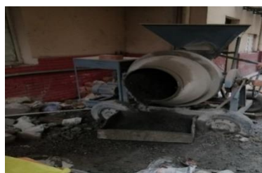
Figure 2. Mixing of concrete
