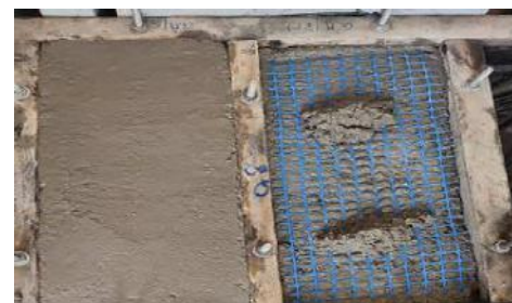
Figure 2. Slab formwork used
