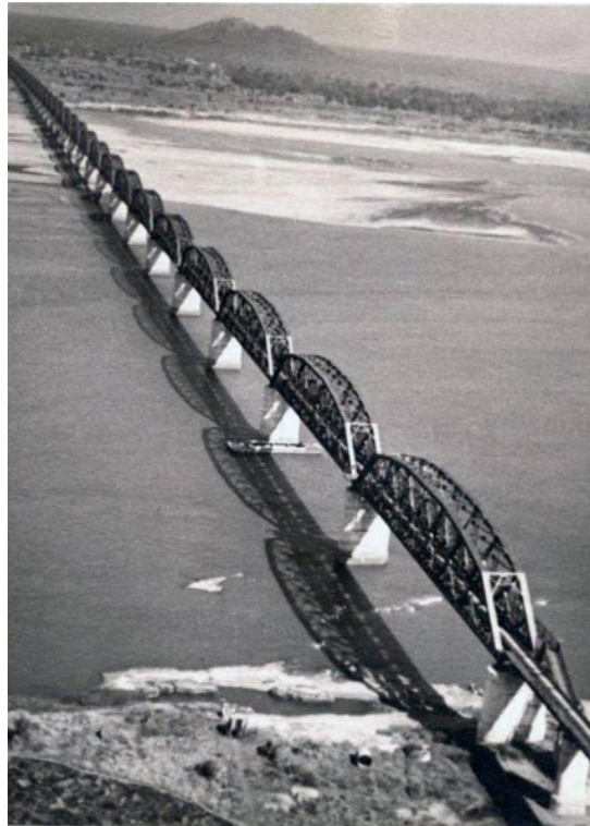
Figure 6. An aerial view of the Dona Ana Bridge, across the Zambezi River. Source: Private archive.
