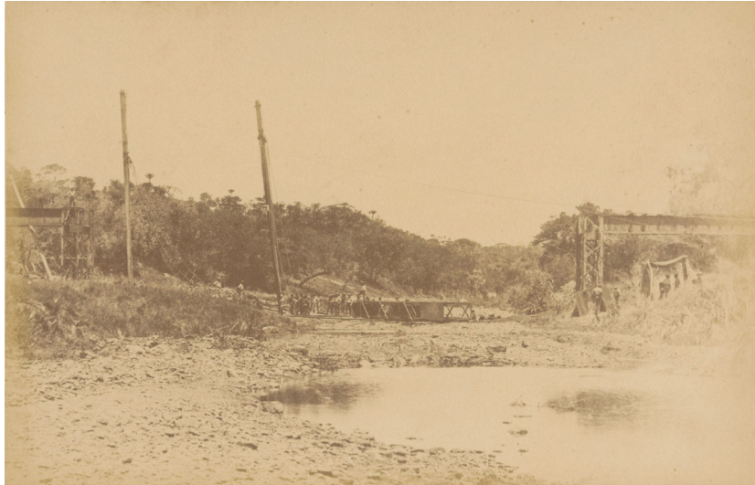
Figure 2. A technical vulnerability in the Lourenço Marques railway is evidenced in the ruins of the Chicongene bridge after the 1889 floods. The Portuguese photographer who took this photo (Romão Pereira) later took another one showing the same bridge rebuilt by Portuguese engineers, stressing how different things were when colonial railways were built by Portuguese experts. Source: Romão Pereira photography of the ruins of the Chicongene bridge after the floods of January 1889, Collecção de Photographias Relativas ao Caminho de Ferro de Lourenço Marques , PT/CPF/CAF/0005/000007, Centro Português de Fotografia (Porto), available at digitarq.cpf.arquivos.pt/details?id=1208376 .
