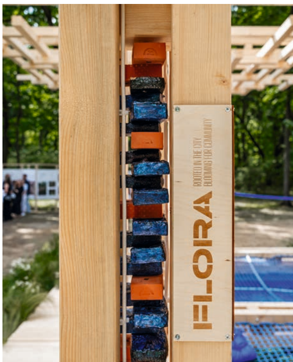
III.3. Mycelium bricks recorded in the structural column of "On the Future Pavilion Construction" - the initiative "We Stand for the Future" - at the Royal Łazienki Museum. Photograph: Artur Brzozowski.
