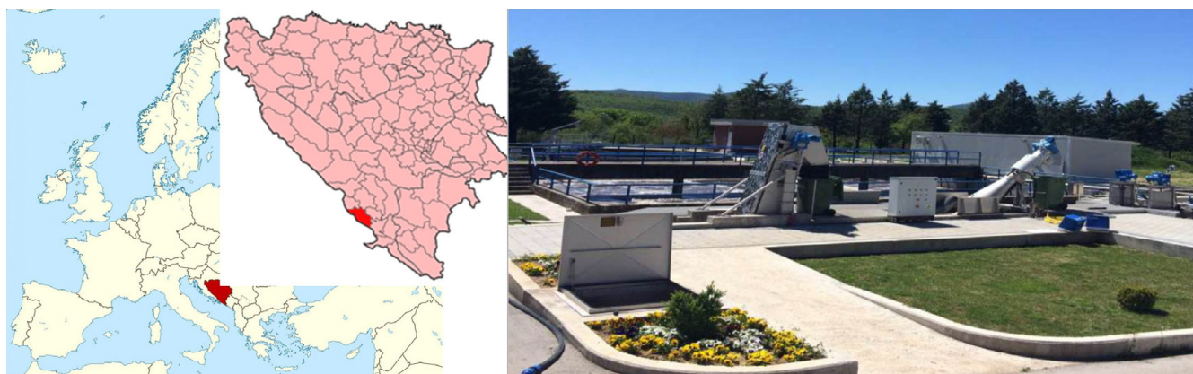
Fig. 1. Location and current state of the WWTP Ljubuški.
