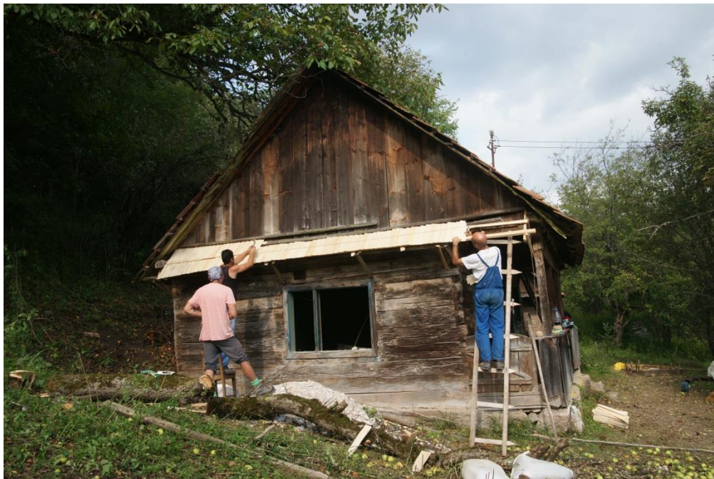
Practicing with wood roofing © Pîrvu Ionică
