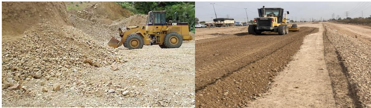
Fig. 4: Shows the natural materials used in the road layers.
