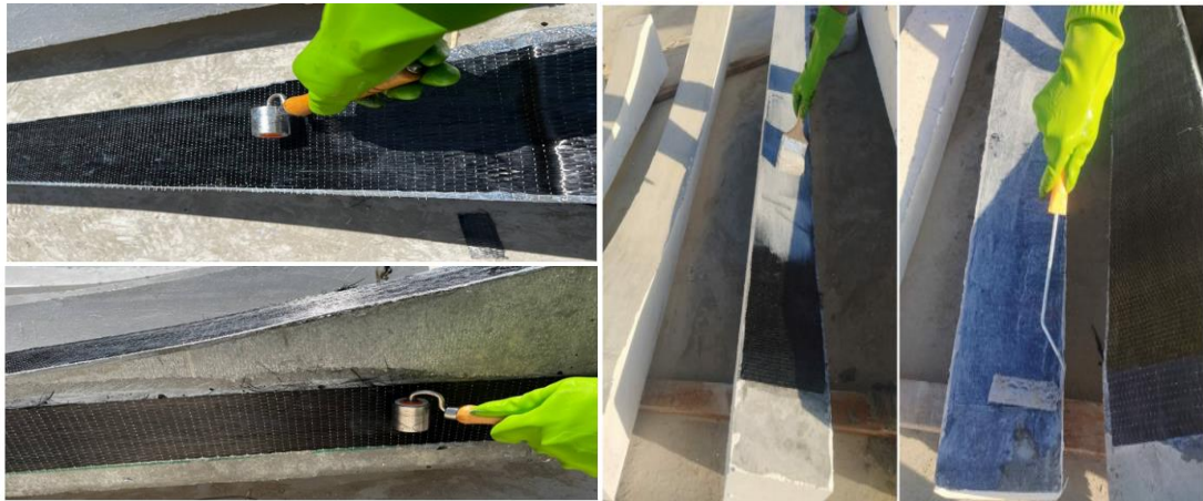
Fig. 6: Application of CFRP sheet.
