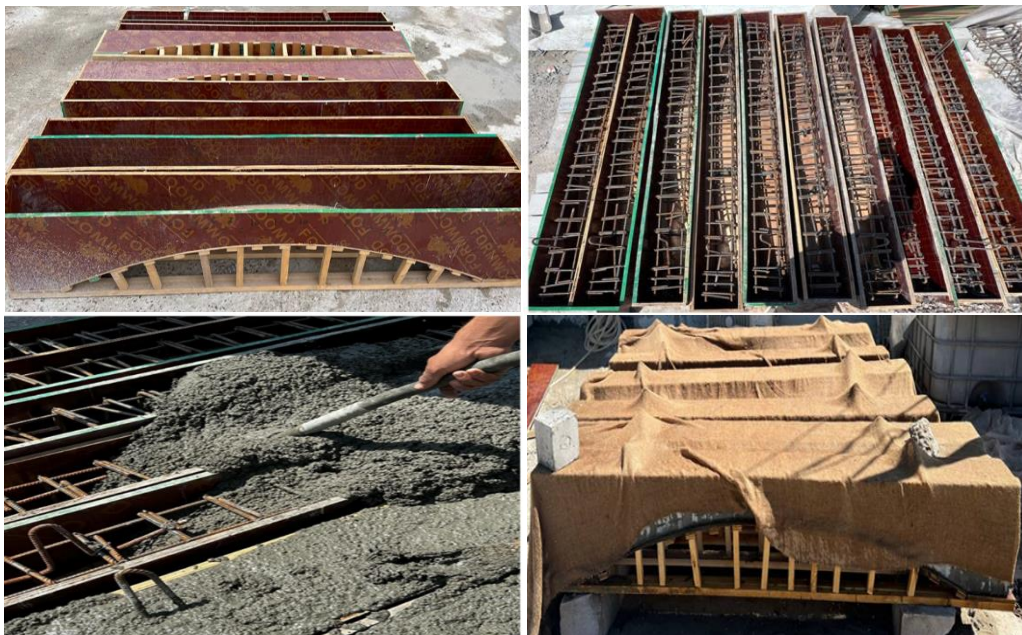
Fig. 3: Casting and curing process.
