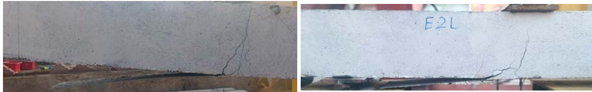
b) De-bonding Mode of Failure (E1L and E2L).
