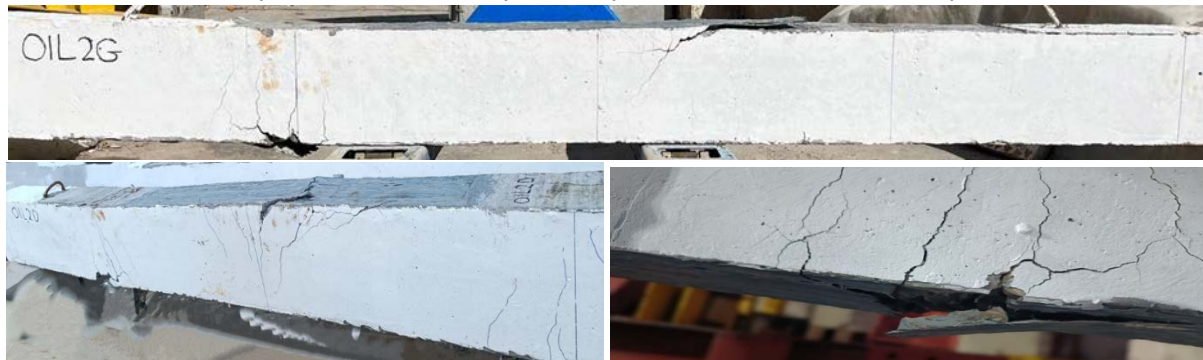
d) CRFP Rupture Mode of Failure (O1L3G, O1L2G, O1LVD and O1L2).
