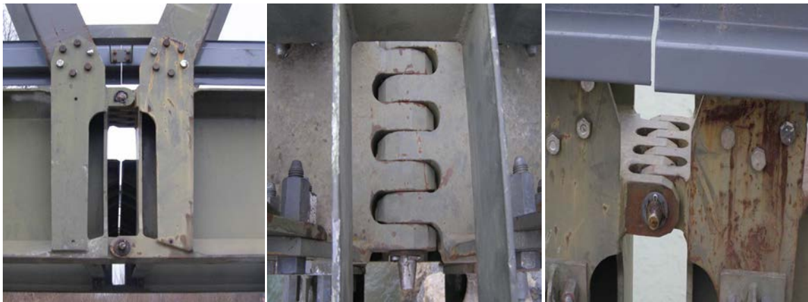
Fig. 4: Pin connection (lock) of the lower chord of the bridge ŽM 60.
