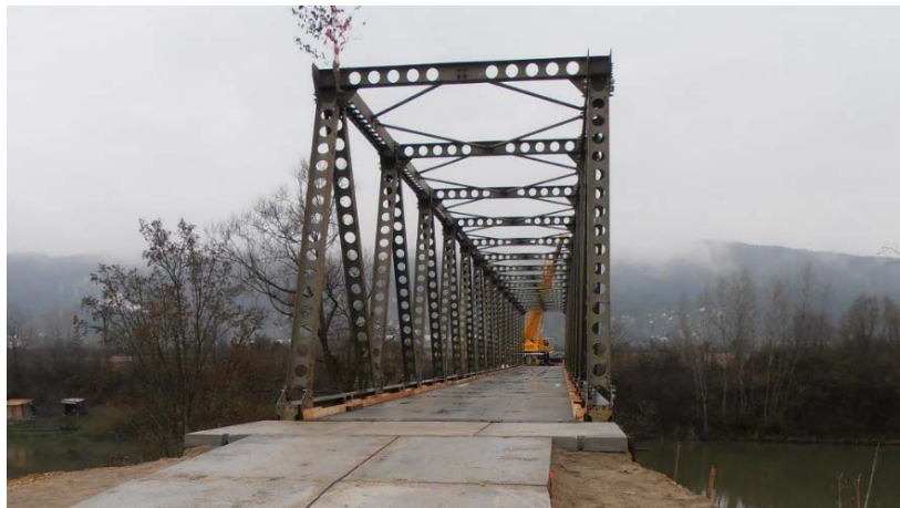
Fig. 16: Temporary bridge ŽM 60 as part of the construction site.
