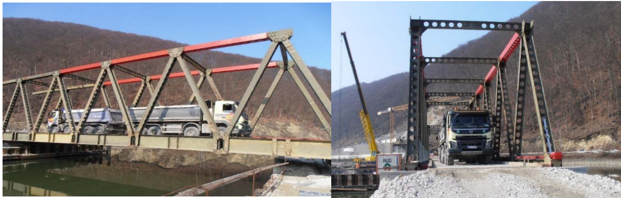
Fig. 9: Load test of ŽM 60 bridge.
