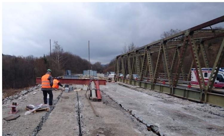
Fig. 12: The damaged bridge during demolition and the temporary bridge ŽM 60 [30].
