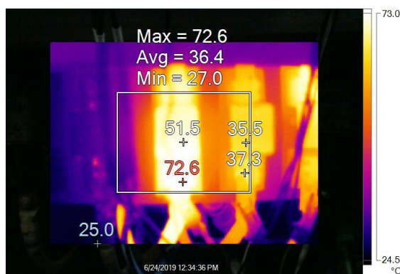
Figure 2: Result of thermal inspection
