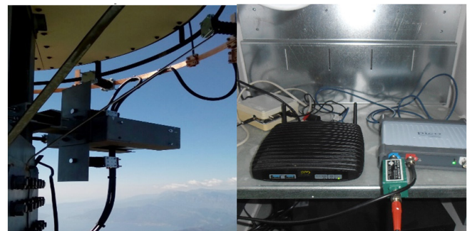
Figure 2: Installation of current transformer (left), monitoring system with industrial computer, GPS receiver and acquisition card (right) [5]
