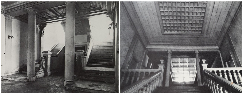
Fig. 6. Left: The imperial staircase on the north end of the ground floor hall ( sofa ) and the Tuscan columns in the hall ( sofa ) [10]. Right: The stairs leading up the second-floor hall ( sofa ) [14].
