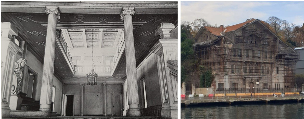
Fig. 7. Left: The two-story hall ( sofa ) between the second and third floors [10]. Right: Italian Embassy summer building in Tarabya [photo by the author].
