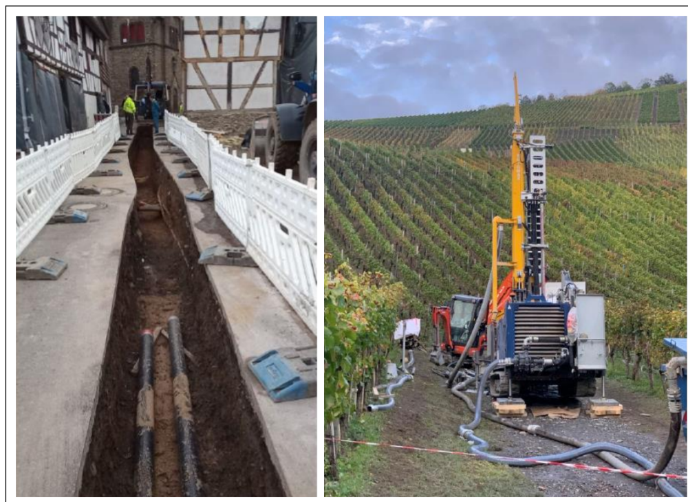
Figure 4 Construction phase of the anergy grid in the city of Rech (left) and exploiting of the borehole heat exchanger field (right) ( Ngahan & Giel 2022 ).
