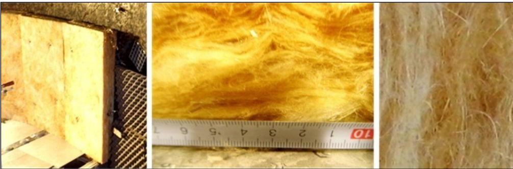
Figure 5 Installation of a 120 mm glass wool plate on the reflected wall and macroscopic open glass fiber surface.
