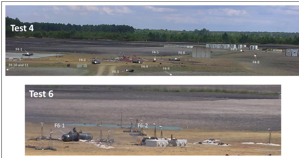
Figure 5 Tests 4 and 6 – Pictures of the experimental test site after the rupture of the tanks with the main fragments.
