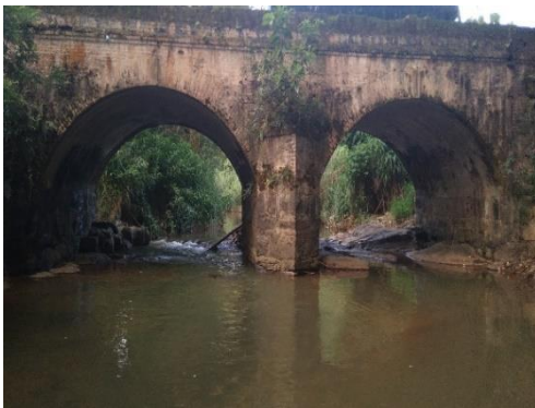
Fig. 1. Nanu Oya arch bridge
