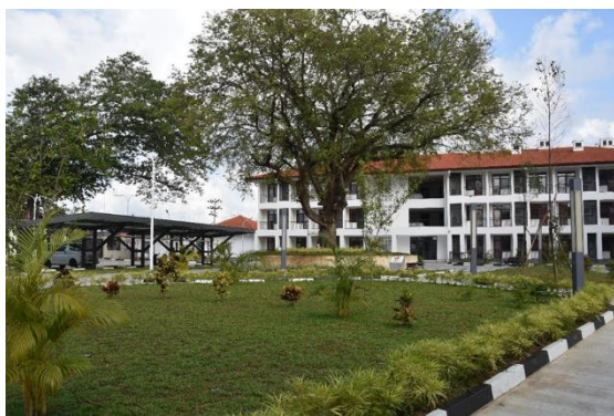
Figure 03: Accommodations area - National Nephrology Specialized Hospital Polonnaruwa - 2022
