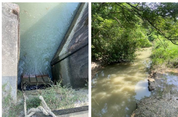
Figure 5: Canal sluice System & local coping Badh (Source: Authors' field survey)
