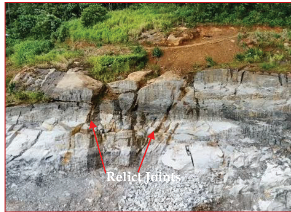
Figure 3 - Highly Jointed Meta-sedimentary Rocks at CEP 3 Cutting Location
