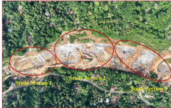
Figure 5 - Study Location (Ch: 9+500 km - Ch: 10+290 km)
