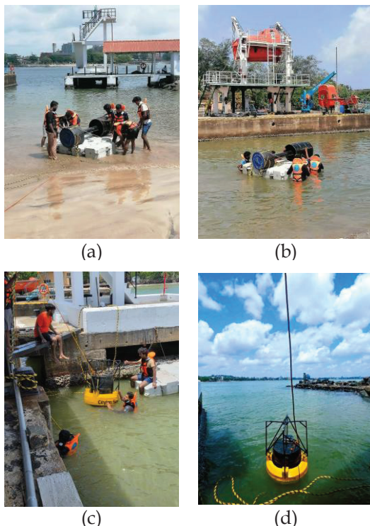
Figure 12 - (a) Assembling device on floating pontoon, (b) Transporting to deployment location, (c) Floater insertion, (d) Successfully deployed Ceylon SURGE WEC
