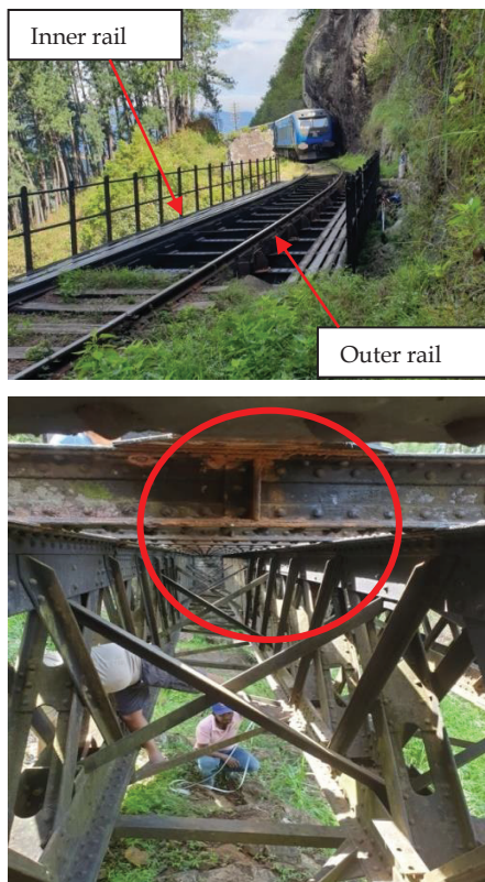
Figure 3 - Two views of the case study bridge I
