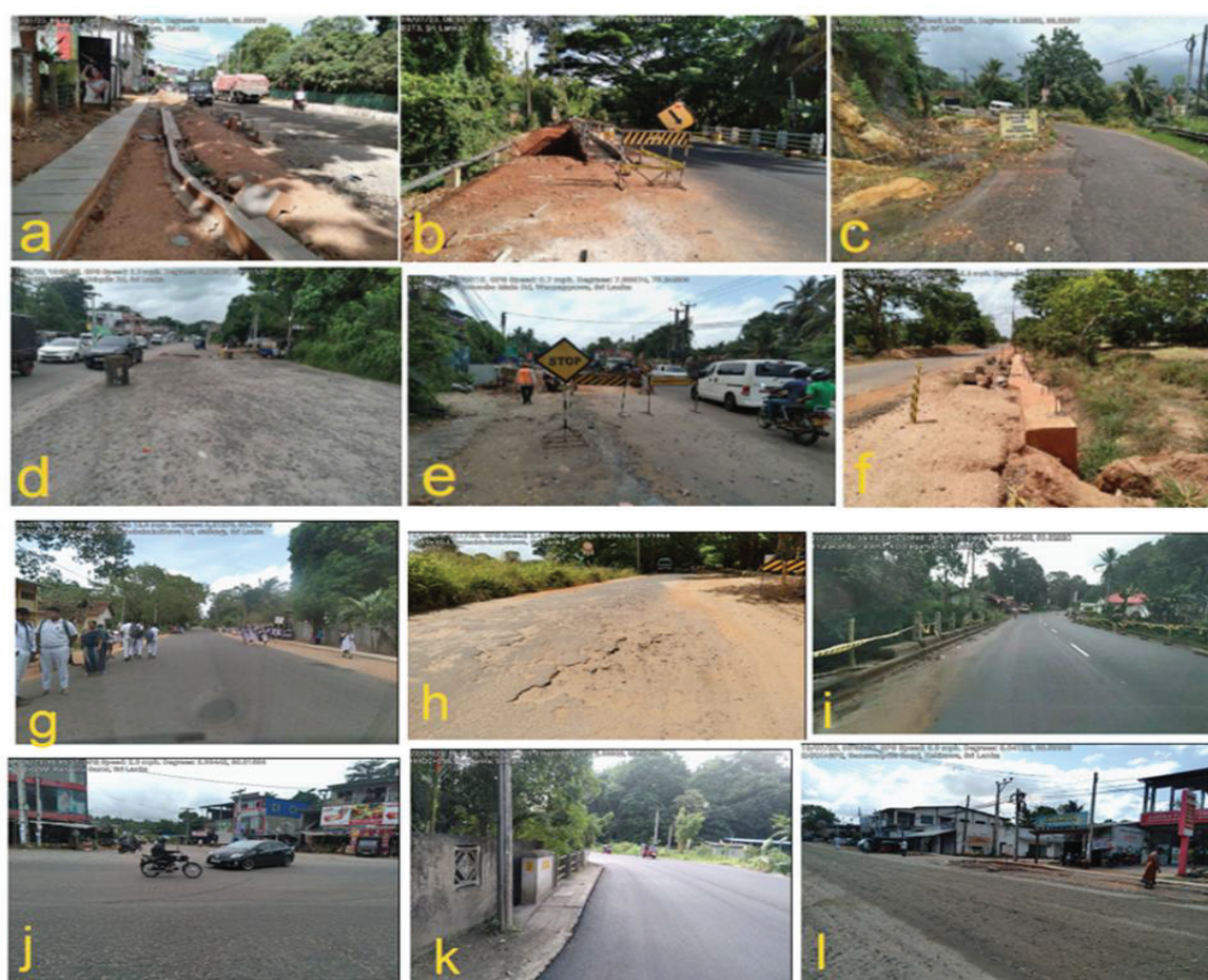
Figure 1 – Sample photographs of audited road sections
