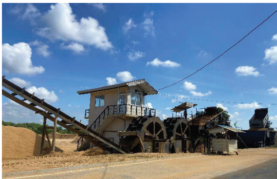
Figure 4 - Sea sand processing machine at Muthurajawela Sea sand yard
