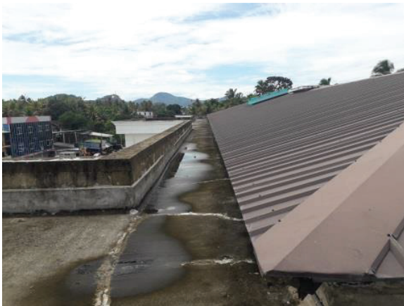
Figure 3 - A photograph of building at Site 2 at Roof level
