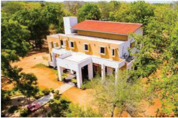
Figure 1(d)- Site 4 - 2 storey office building having a total floor area of 1135m 2
