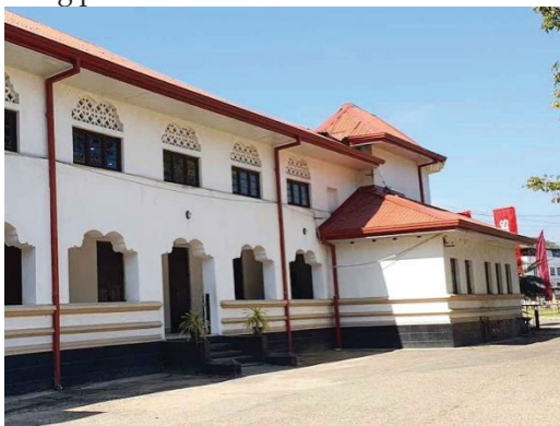
Figure 2 - Premixed parking areas of the Site 1
