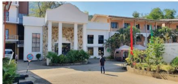
Figure 1(a)- Site 1- 3 storey office building having a total floor area of 5440 m 2
