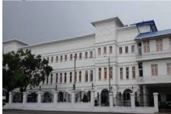
Figure 1(c)- Site 3 -3 storey office building having a total floor area of 1180m 2
