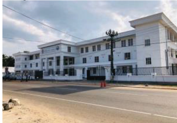
Figure 1(b)- Site 2-3 storey office building having a total floor area of 2361m 2
