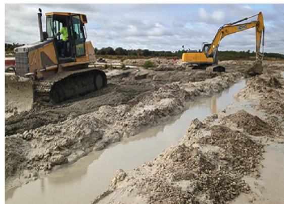
Figure 1 - Trenching under bentonite slurry in Miller pump station in Naples [11]
