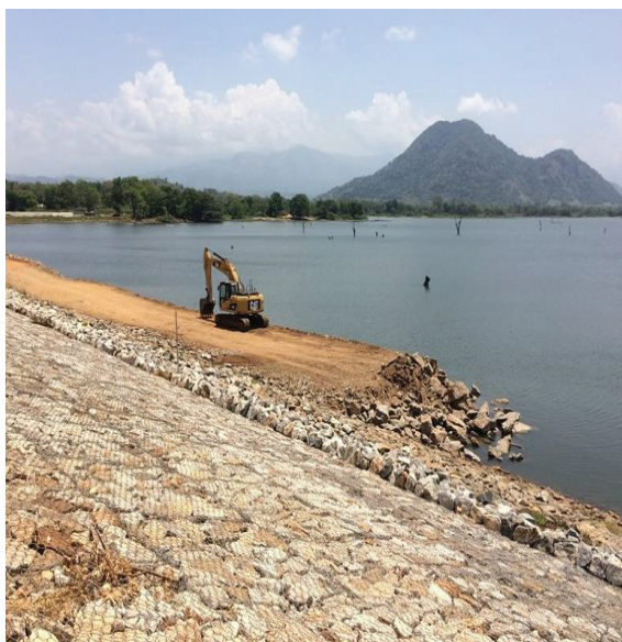
Figure 13 - Upstream Loading in Handapanagala Reservoir
