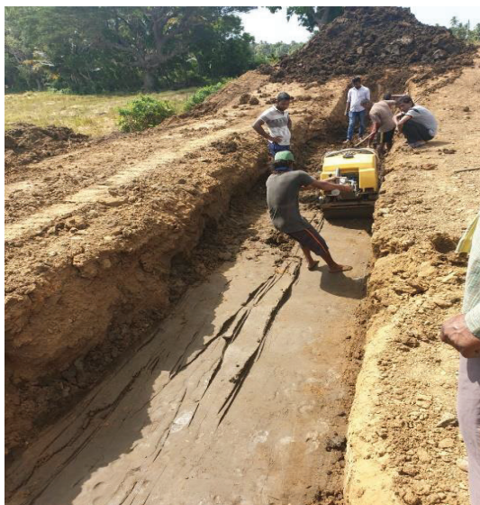
Figure 12 - Clay Core Placement and Compaction
