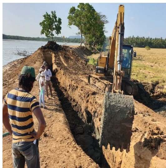
Figure 11 - Clay Core Trench Excavation in Debarawewa Reservoir
