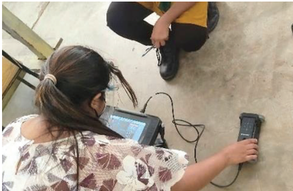
Figure 4 - Cover Meter Test on a Reinforced Concrete Slab
