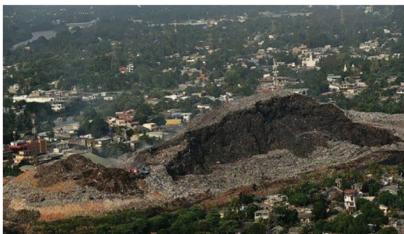
Figure 1 – Meethotamulla Dump Site after Failure
