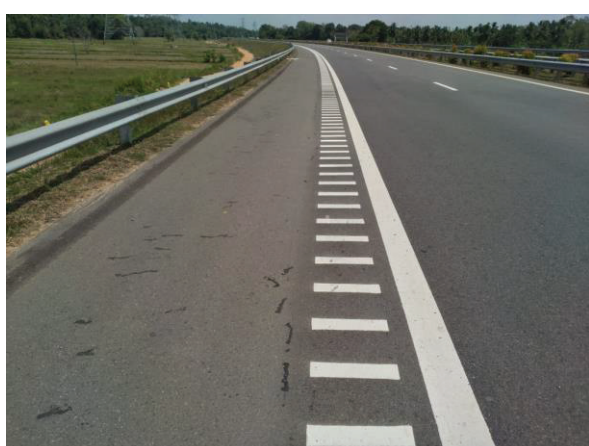
Figure 2 - Shoulder Rumble Strips Installed on the Central Expressway (CH 39+600 LHS)
