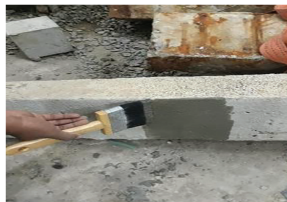
Figure 7 - Application of Xypex as Retrofitting Material
