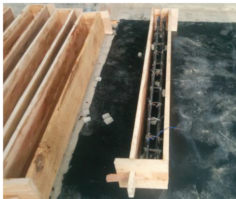
Figure 2 - Reinforcement and Formwork of Test Specimens
