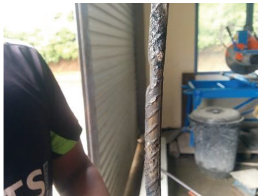
Figure 6 - Corroded Reinforcement Bar Extracted from Specimen
