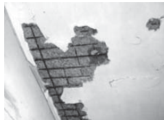
Damaged slab
