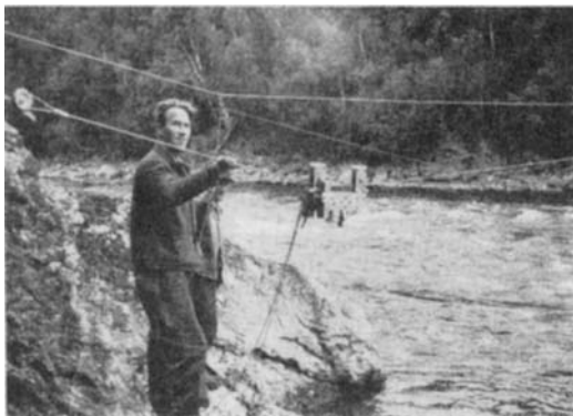
Fig. 3. Rope-way across a rapid, for the placing of explosive charges at the river bottom.
