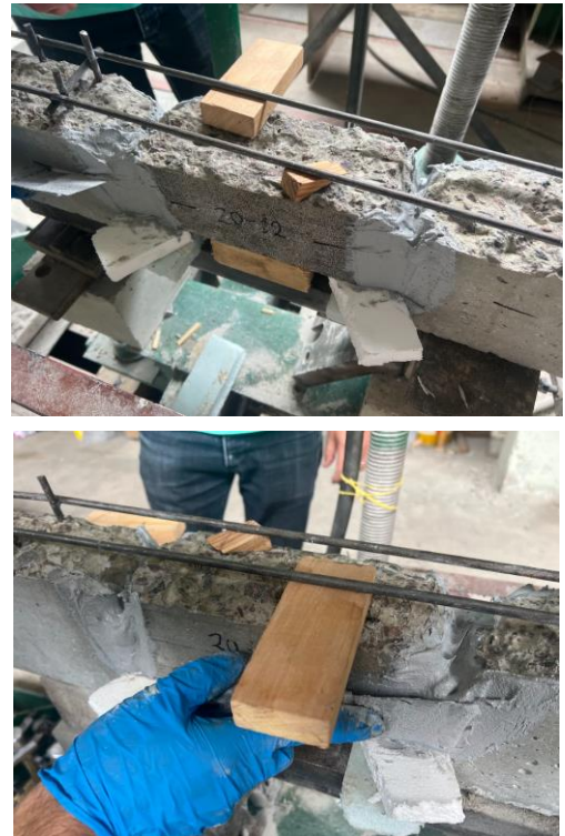
Fig. 11. Pressing in the epoxy adhesive and allowing it to cure
