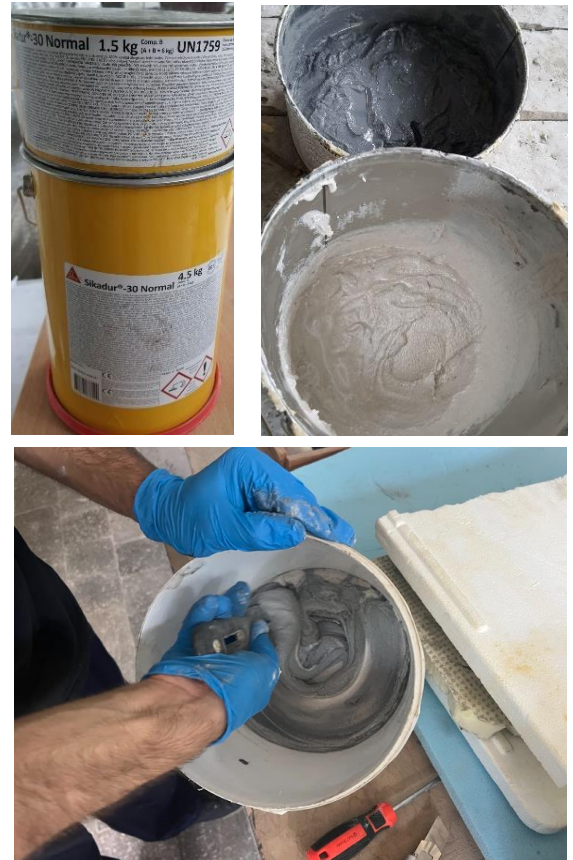
Fig. 7. View of the damaged area of the RC beam
