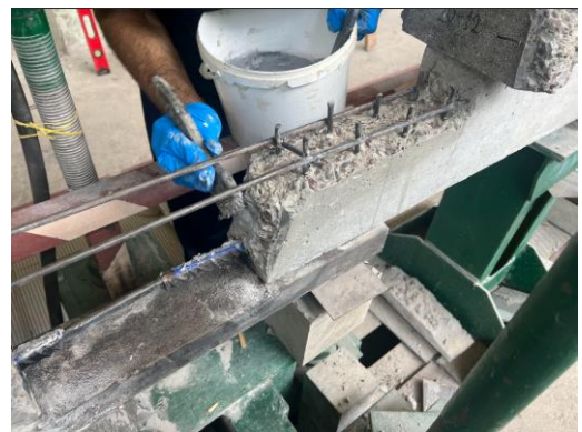
Fig. 8. Priming the surface with epoxy adhesive
