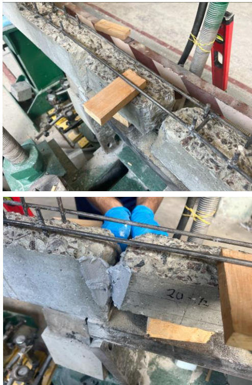
Fig. 10. Positioning the insert in the designed position and securing it
