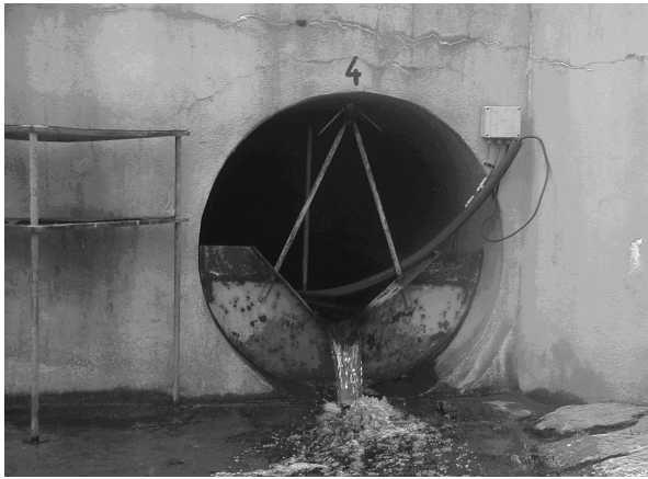
Fig. 2. Discharge gauging profile on the Teply Brook catchment.
