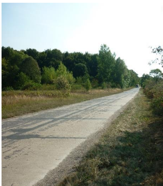
Figure 1. View of the surface of roads on which acceleration values were measured - straight
