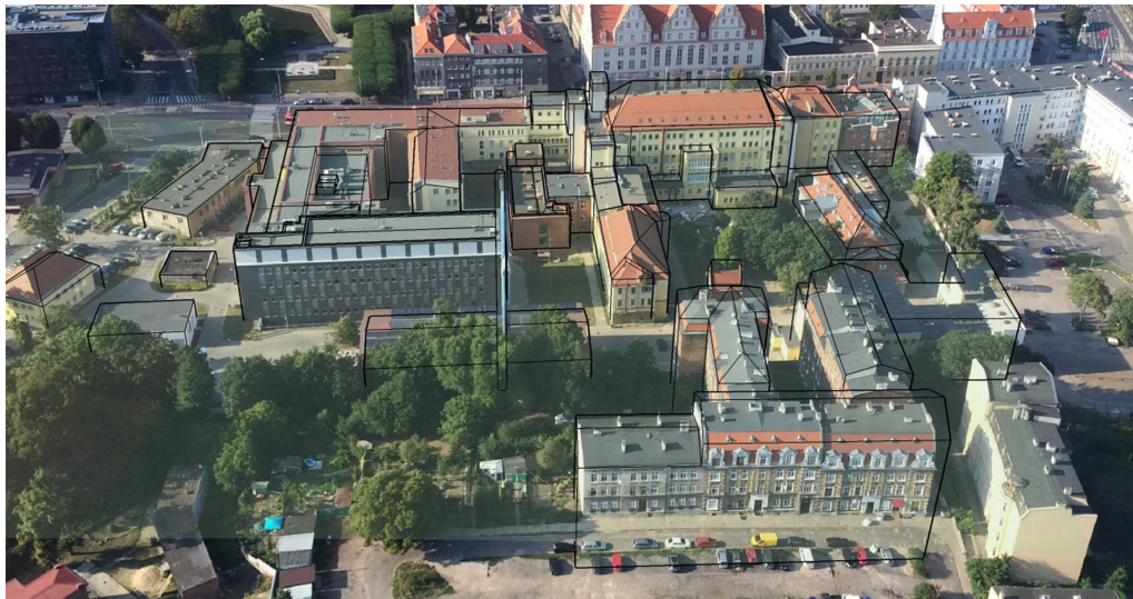
Fig. 31. The Copernicus Hospital in Gdansk – photogrammetric comparison between the model and an aerial photograph [22].
