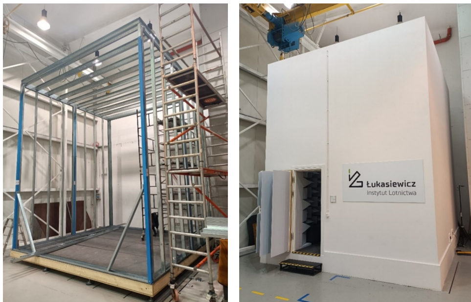
Fig. 1. The anechoic chamber at Ł-ILOT during construction and after completion.
