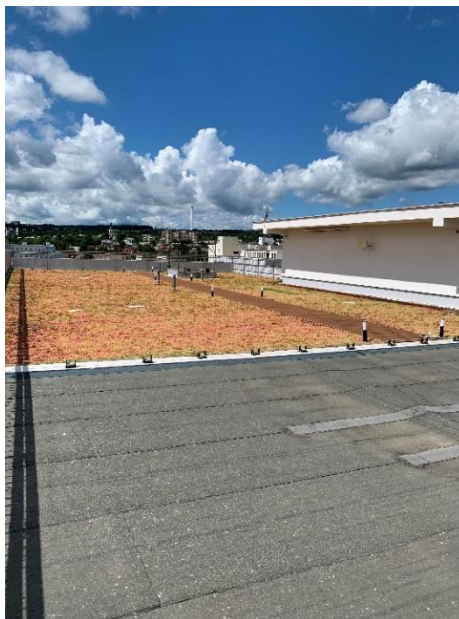
Figure 1: View of the main TUKE building rooftop, illustrating the adjacent green-roof section and the asphalt-covered surface
