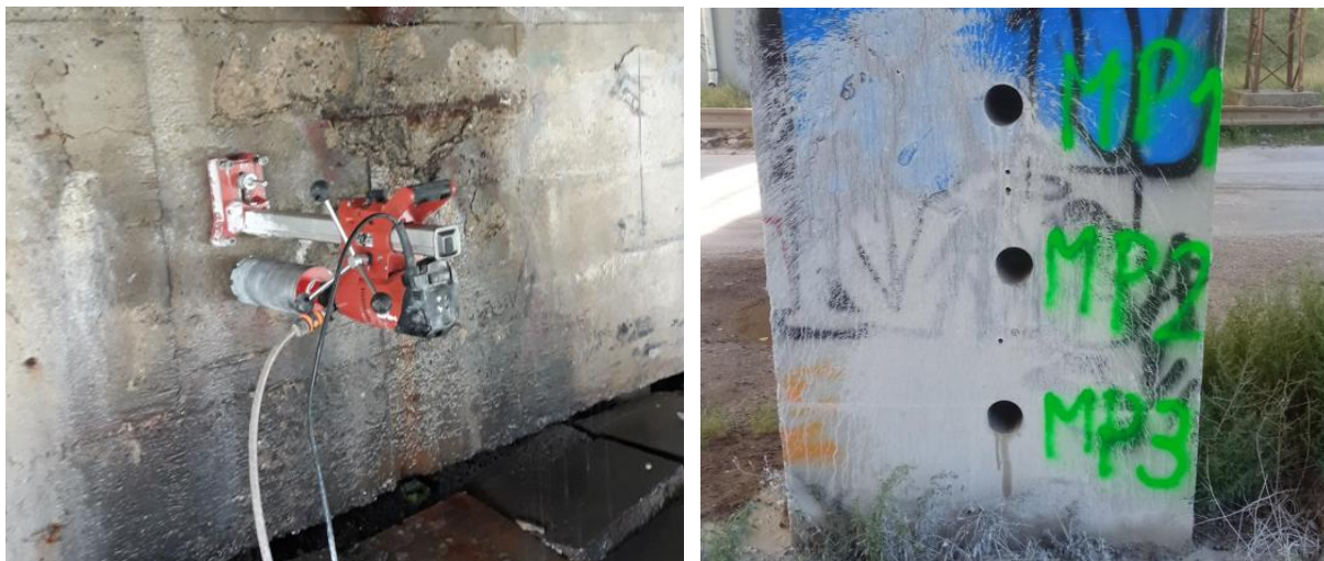
Figure 1: The process of core drilling the and a view of the holes after the drill bits have been removed
