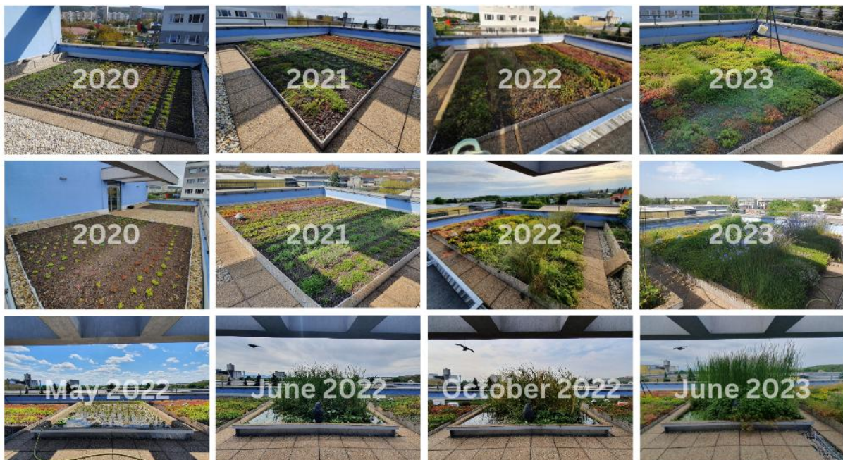
Figure 2: Development of vegetation cover on an extensive green roof and a wetland roof from installation to full coverage. The comparison highlights the considerably faster establishment of wetland vegetation under stable water availability [Source: Author]
