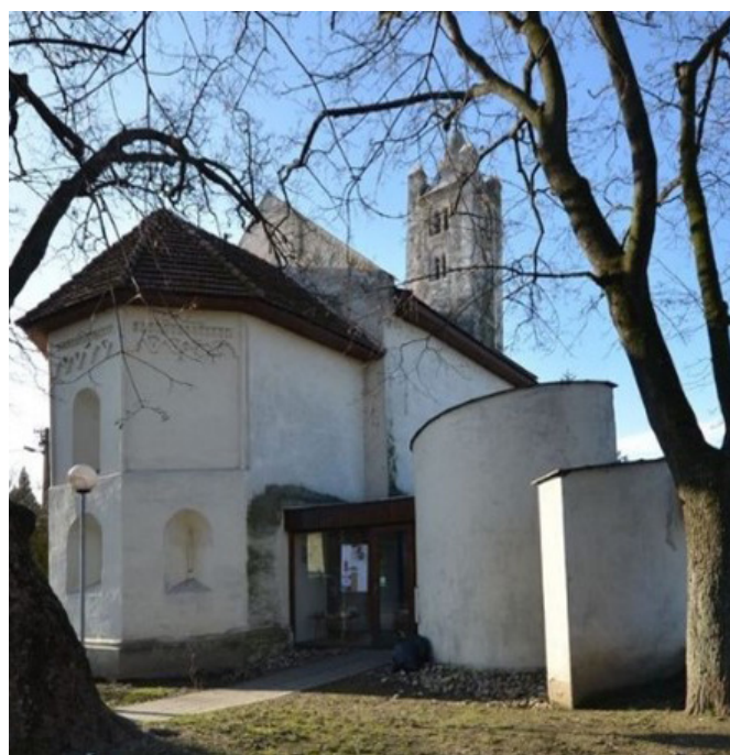
Fig. 1 Church in Hamuliakovo (Slovakia) – Annex of sacristy to the presbytery. Source: https://apsida.sk/c/2/hamuliakovo
